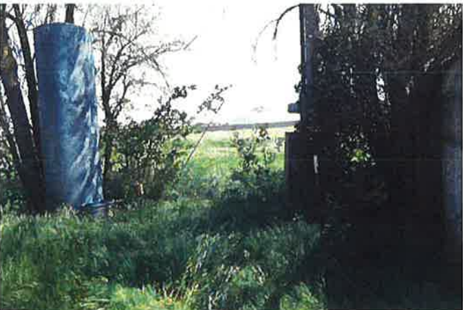
Photo 29 – APN-014 rear of south house
