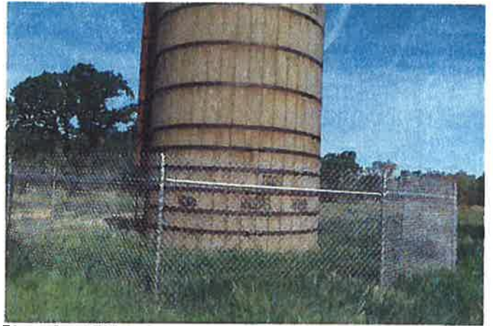
Photo 8 – APN-015 water tower
