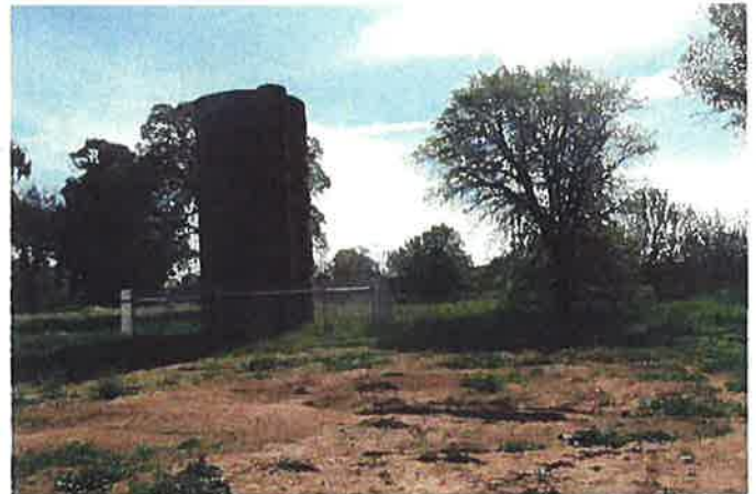
Photo 4 – APN -015 water tower
