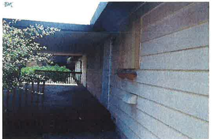
Photo 30 – APN-014 rear of north house
