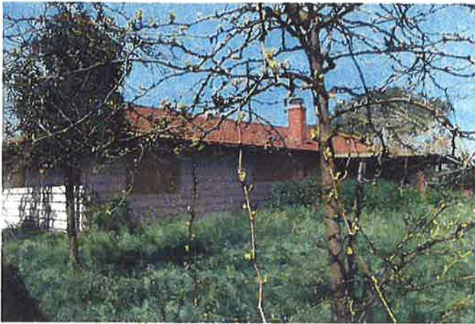
Photo 31 – APN-014 rear of north house
