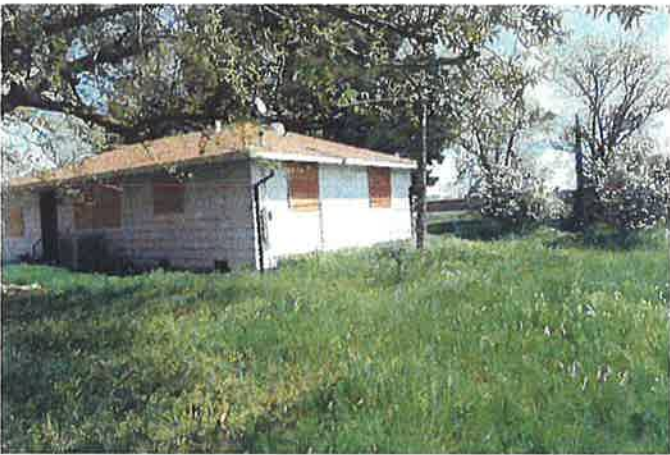
Photo 21 – APN – 014 south house
