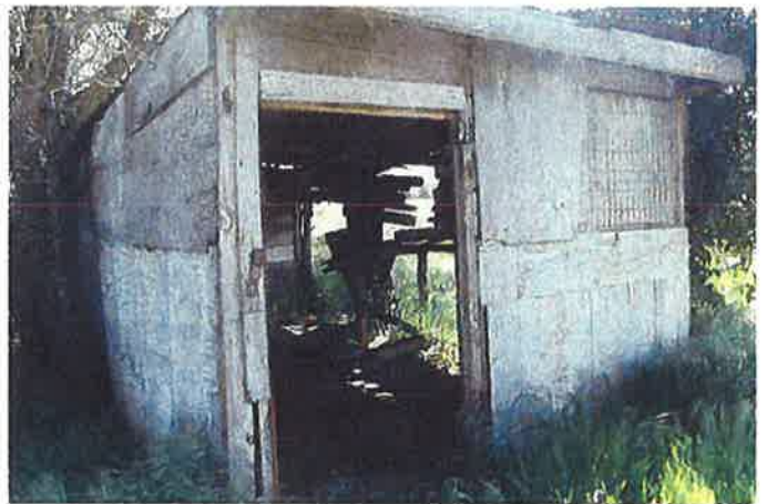
Photo 22 – APN – 014 shed behind south house
