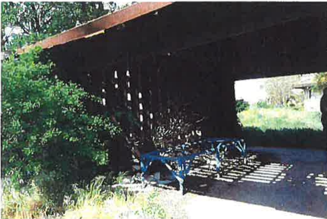
Photo 27 – APN-014 front of middle house
