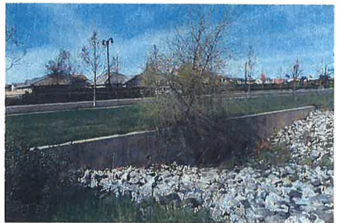
Photo 12 – APN -011 culvert under Big Horn Boulevard
