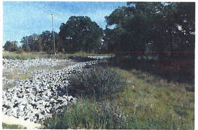
Photo 10 – APN -011, drainage creek
