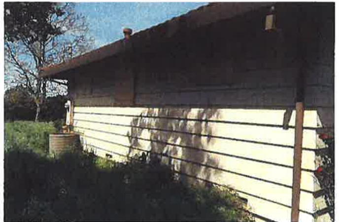
Photo 28 – APN-014 side of north house
